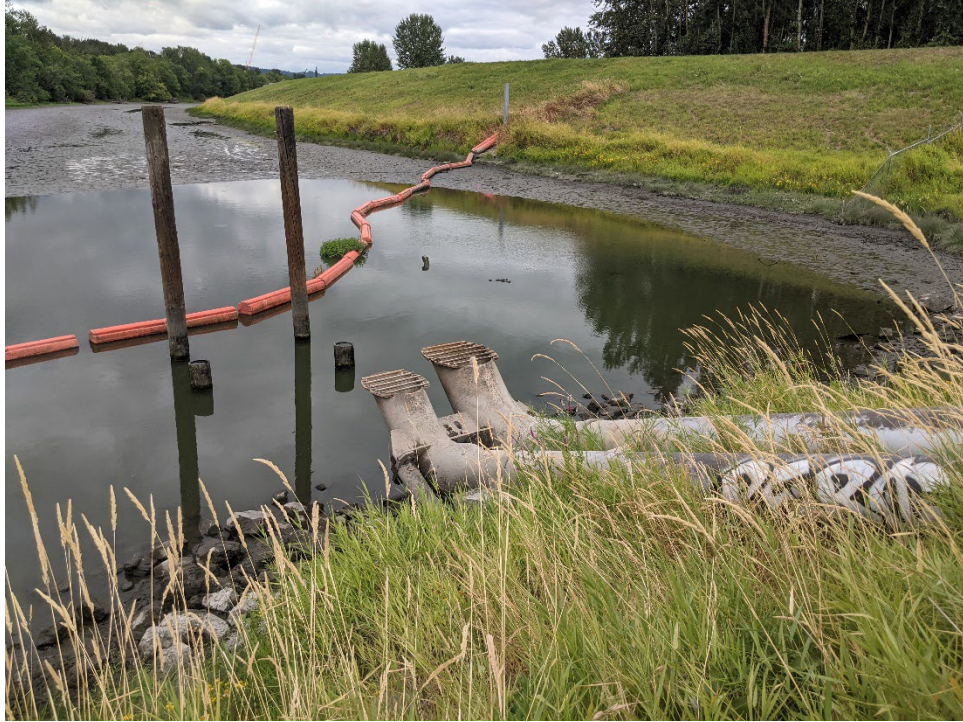
Photo 7. PIR Discharge into Columbia Slough
