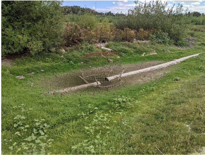
Photo 11. Vanport Wetlands - Beaver Deceiver Structure
